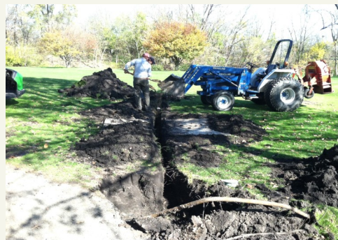
Repairing a Drainage tile by Number Two green
